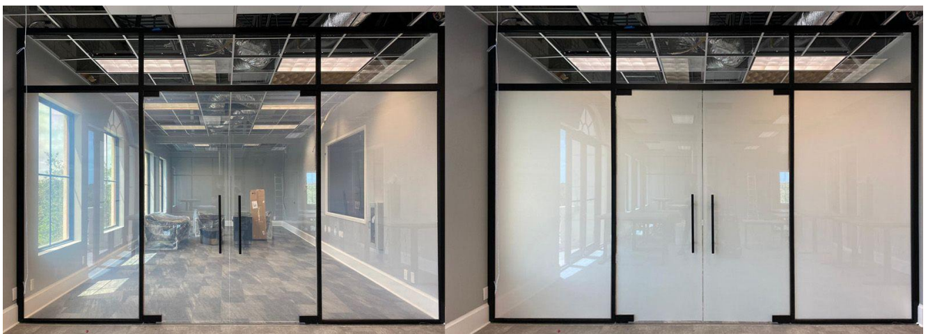
Figure 3 electrochromic glasses allow you to control the amount of light that passes through them, becoming transparent or opaque
