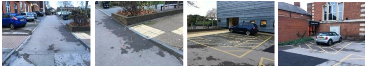
Figure (3): Accessible Car Park and Ramps in Front of Each Entrance in the Building{17} (goldsmith, university of london,
