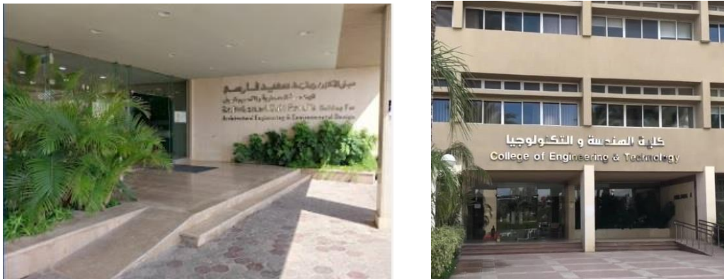
Figure (18): Main Entrance of Engineering Building with clear doors, steps, ramp, and handrails
