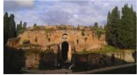
Figure 1. The Mausoleum of Augustus in 2016 before restoration [33]
