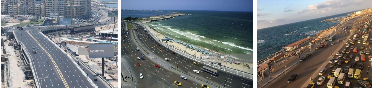
Figure 5 Sidi-Gaber bridge (masrawy.com, 2020), the cornice street development start and its capacity after five years (gettyimages.co.uk, 2020; wikimedia.org, 2020)
